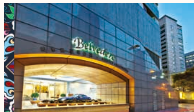
Shanghai Belvedere Service Apartment
