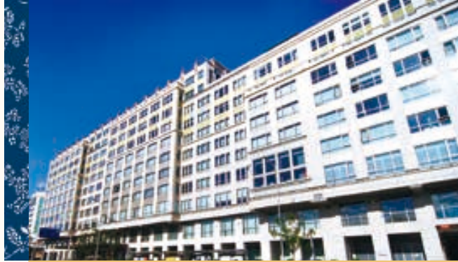
Beijing Xin Yi Garden Phase III Commercial Building
