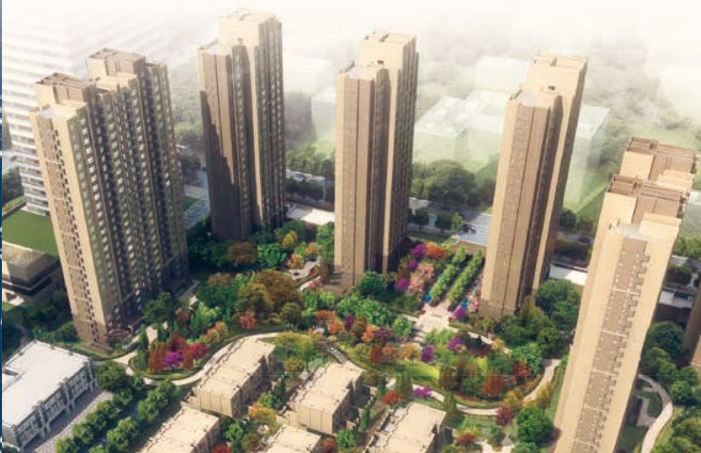
Perspective of the residential portion of Langfang New World Centre "Victoria Garden"
