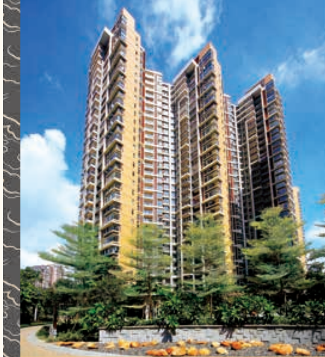
Guangzhou New World Oriental Garden Phase III “The Radiance”
