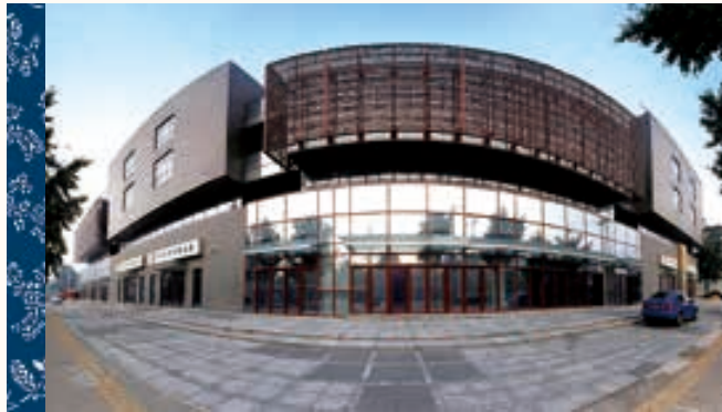
Beijing Yanjing Building
