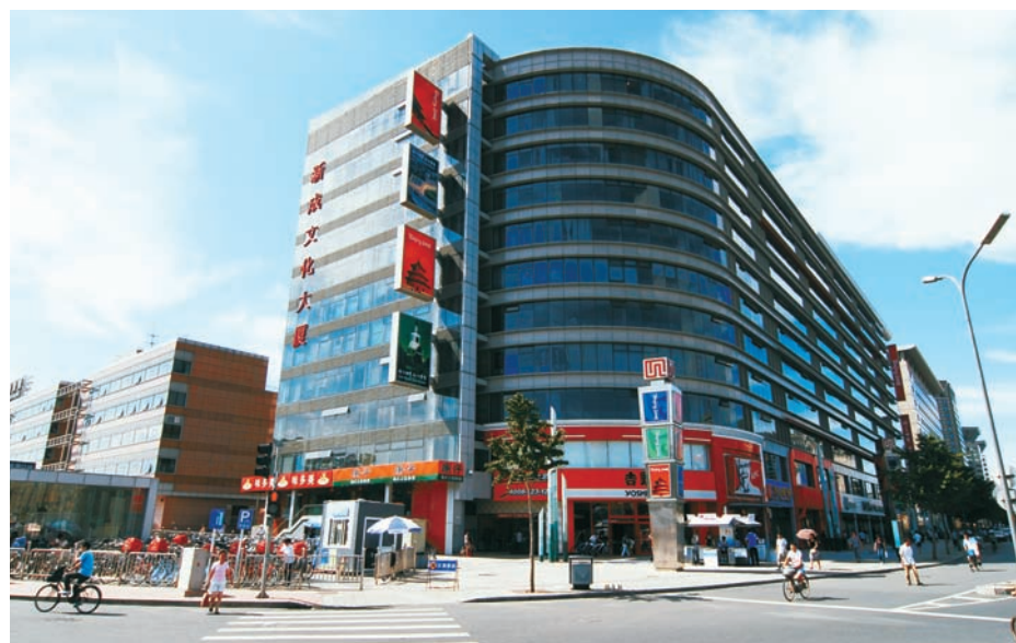
Beijing Xin Cheng Commercial Building
