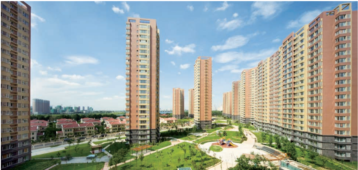
Shenyang New World Garden Phase I Riverridge Heights
